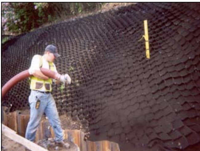
Application of compost blanket roadside County Road 41 in Carver County.
