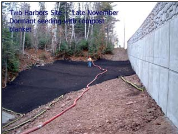
Dormant seeding a compost blanket at a Two Harbors site in late November.
