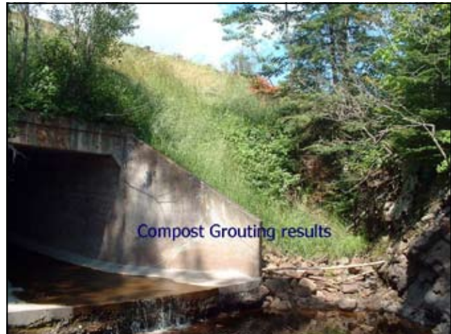
Highway 61 roadside after application of compost grouting.
