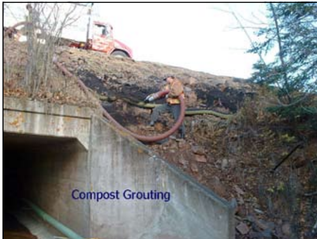
Compost grouting on Highway 61.
