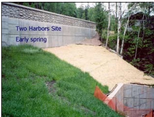
The same Two Harbors site in early spring. Compost blanket on left, seeded straw mat on right.
