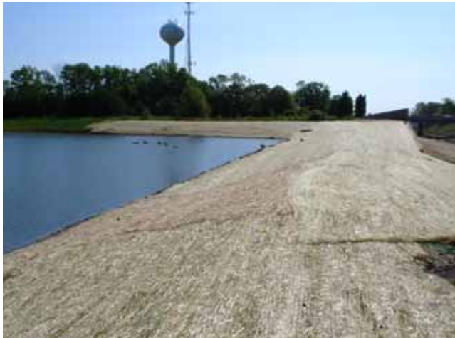
Erosion control blanket stabilizes pond slopes.
