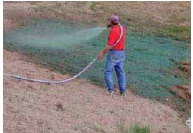
Hydroseeding promotes the rapid growth of vegetation and prevents erosion.
